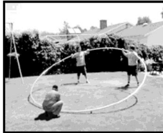
5 Bring both sides of the circle firmly together and secure with small set-screw. A 3rd person may be required to hold the other end down.
